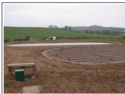
Phase 1, which consisted of installing the reed-bed system to cover the day to day operation of the Hotel, was completed in November 2011. The next phase will be the installation of the large pond with its constructed outlet. In the meantime the additional wastewater created during the major events is partially fed to the reed-bed and tankered away.
